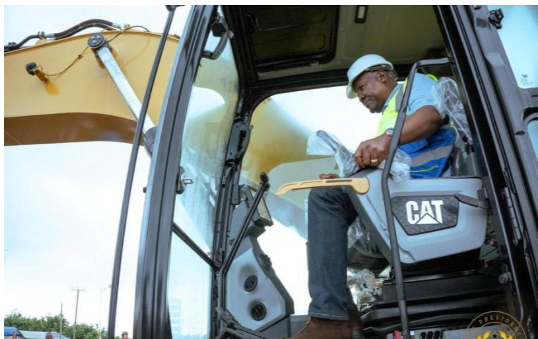
Sod-cutting of Dodowa-Afiinya Road
