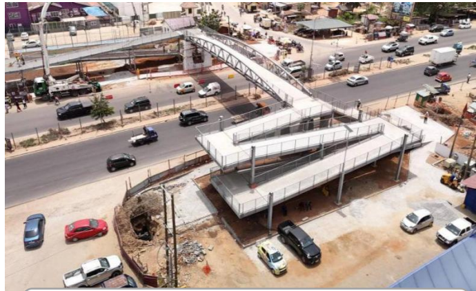
Tetegu Pedestrian Bridge
