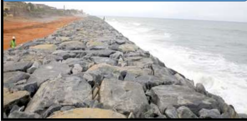
The Completed Revetment Wall with Lateritic Backfilling at Amanful K
